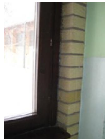
Picture 7. Inner brick facade siding
