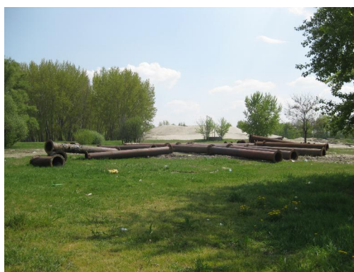
Figure 2. Current state- Rusty pipes
