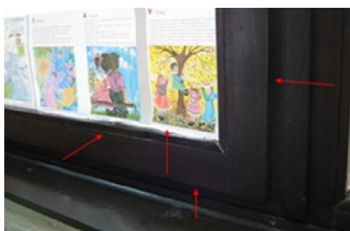
Figure 2. Window critical points
